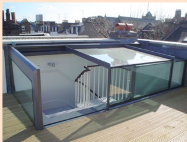
Fig. C8 Box Rooflight Installed
